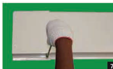
7 Tighten the M5 bolts (2 pcs.)
