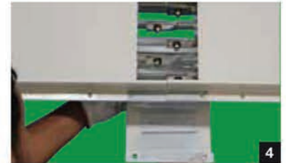
4 Install the rear joint cover with phase barrier.
