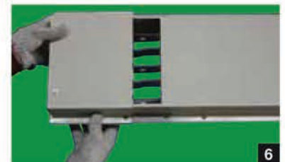
6 Install the end closer at the end of route.
