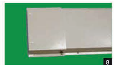
8 Completed end closer joint.
