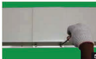
5 Install the front joint cover and tighten the M5 bolts (4 pcs.)
