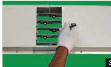
3 Tighten the joint bolts with the torque wrench. It clicks at the regular torque. (130kgf. cm)
